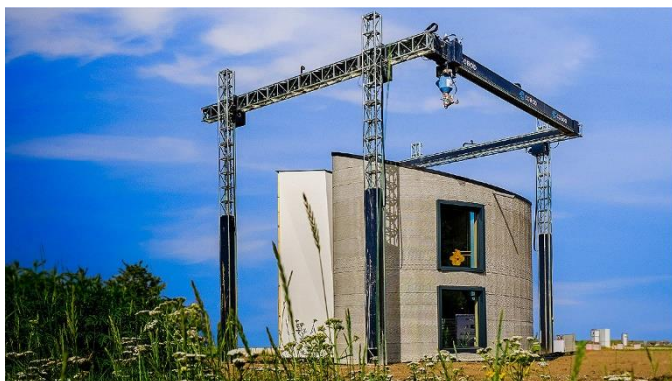
3D print of house https://ww3.rics.org/uk/en/modus/built-environment/construction/cobod-machines-3d-printing-homes.html
