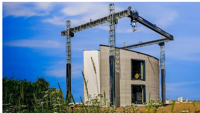
Impression 3D d'une maison https://ww3.rics.org/uk/en/modus/built-environment/construction/cobod-machines-3d-printing-homes.html
